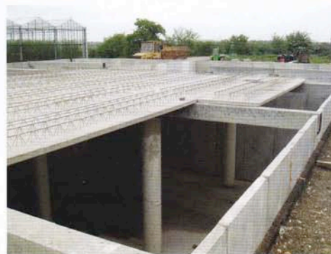
Above: Guy and Wright chop up approximately 50 tonnes of organic waste daily to go into its underground anaerobic digesters (below)
